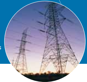
Electricity power lines
