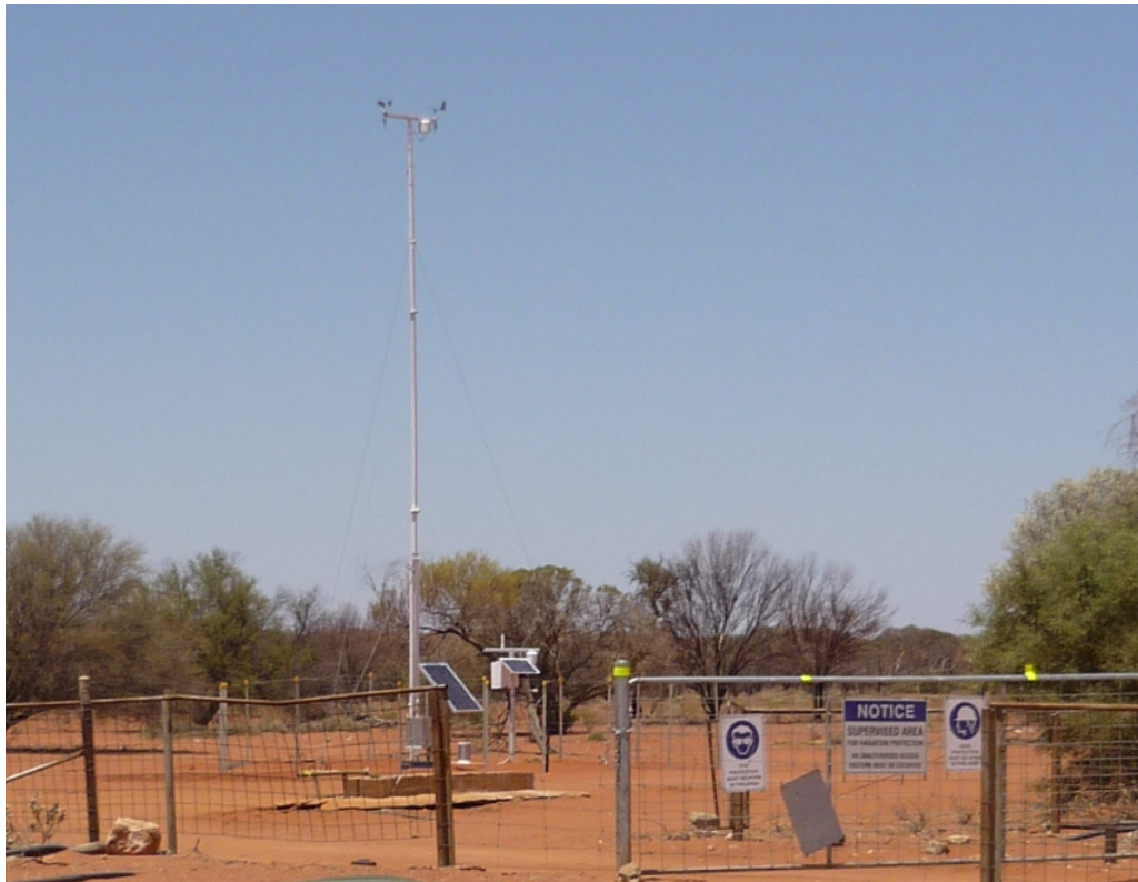
Solar/battery powered weather station collecting site meteorological data
