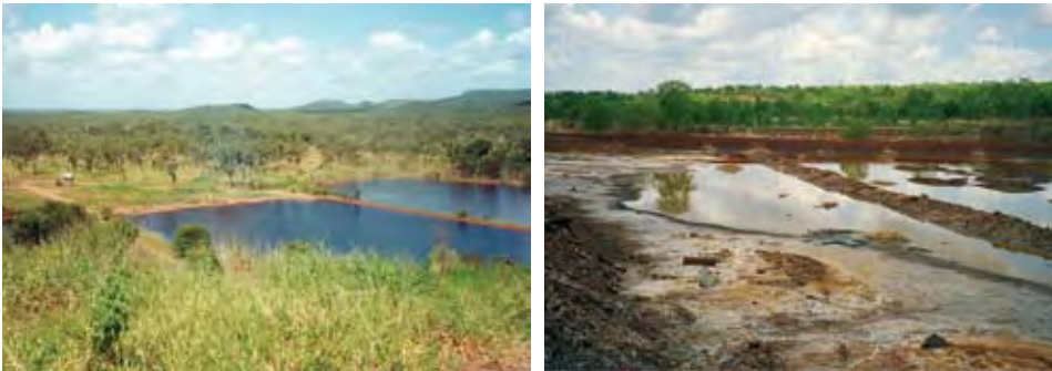
Figure 18: Wetland constructed to polish seepage from a covered waste rock pile. Left panel shows the wetland during initial years of neutral drainage. The right panel shows the wetland after it was overwhelmed and rendered ineffective by breakthrough of highly acidic and metal rich seepage.
