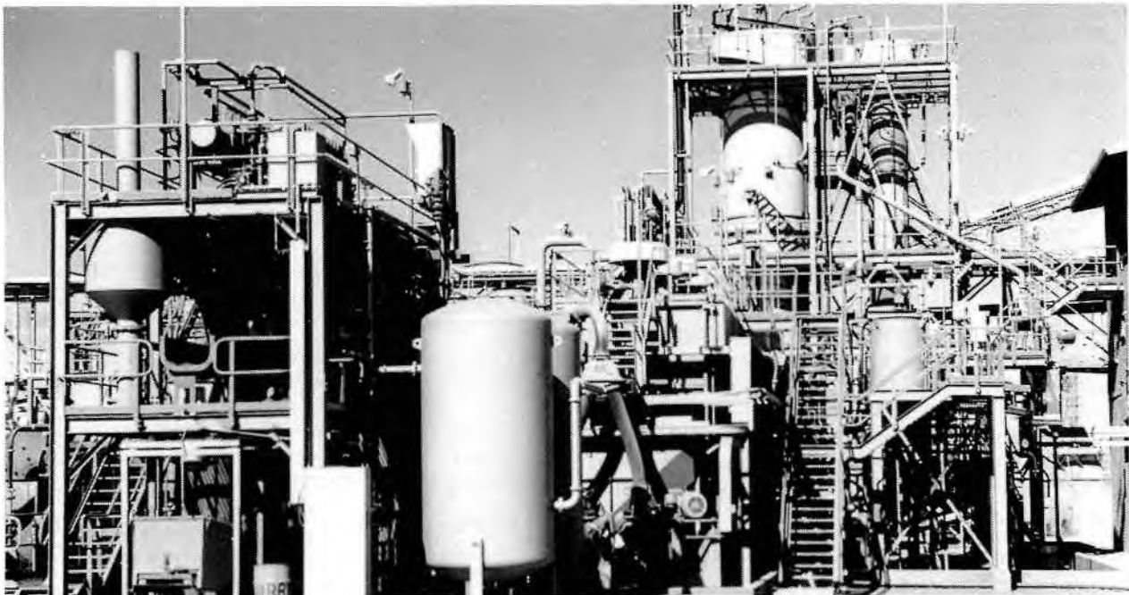
The sulphide ore processing plant at the Harbour Lights Gold Mine.
