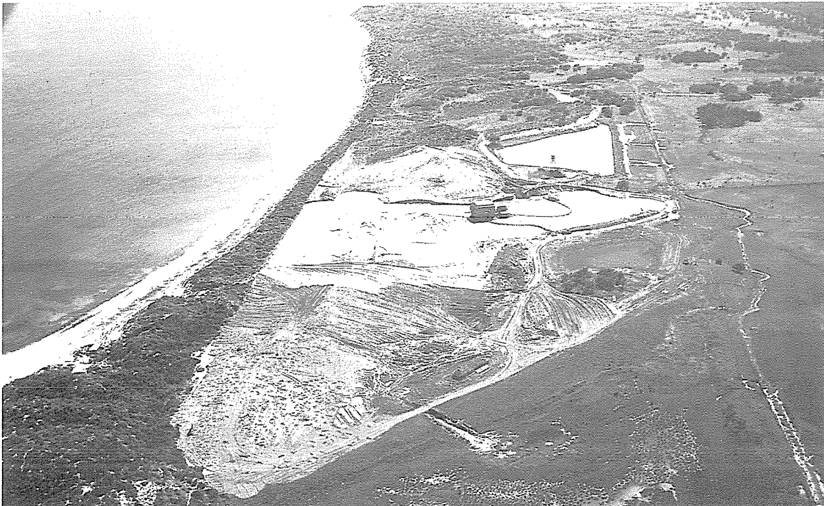
Dredging operations, Minninup, W.A. 1986-87.
