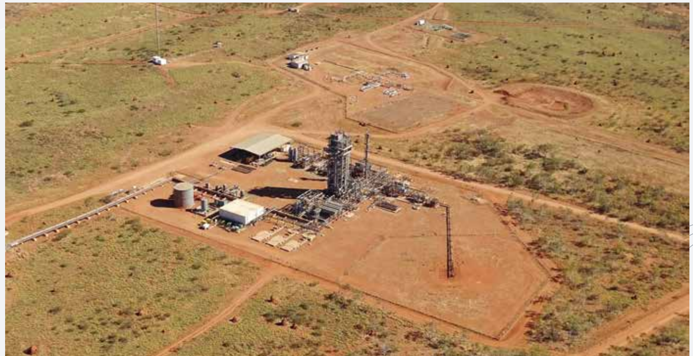
Site of WA's largest gas storage facility. Photo: DDG Tubridgi
