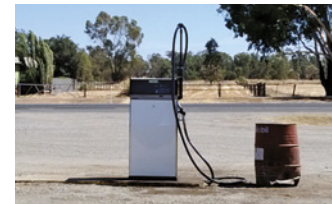
Old drums filled with concrete used as impact protection
