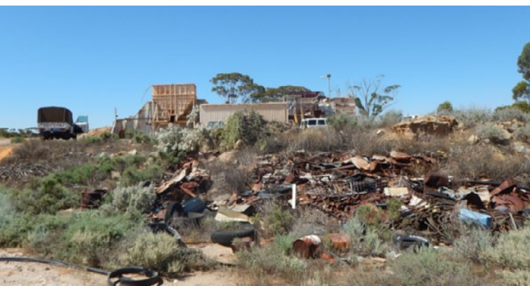
Plant and scrap material before the rehabilitation works in February 2016
