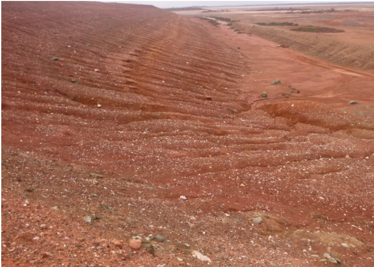
PHOTO 1: EROSION OF TSF EMBANKMENT
