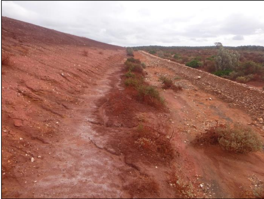
PHOTO 4 : NORTHERN EMBANKMENT TOE EROSION
