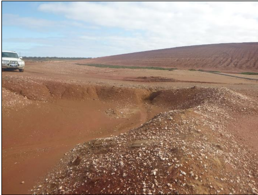
PHOTO 12 : BLOCKED DRAIN ADJACENT TO POND
