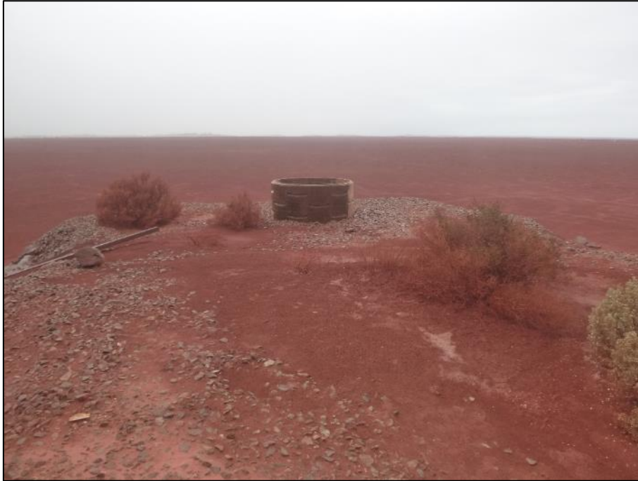
PHOTO 8 : CAUSEWAY AND DECANT TOWER
