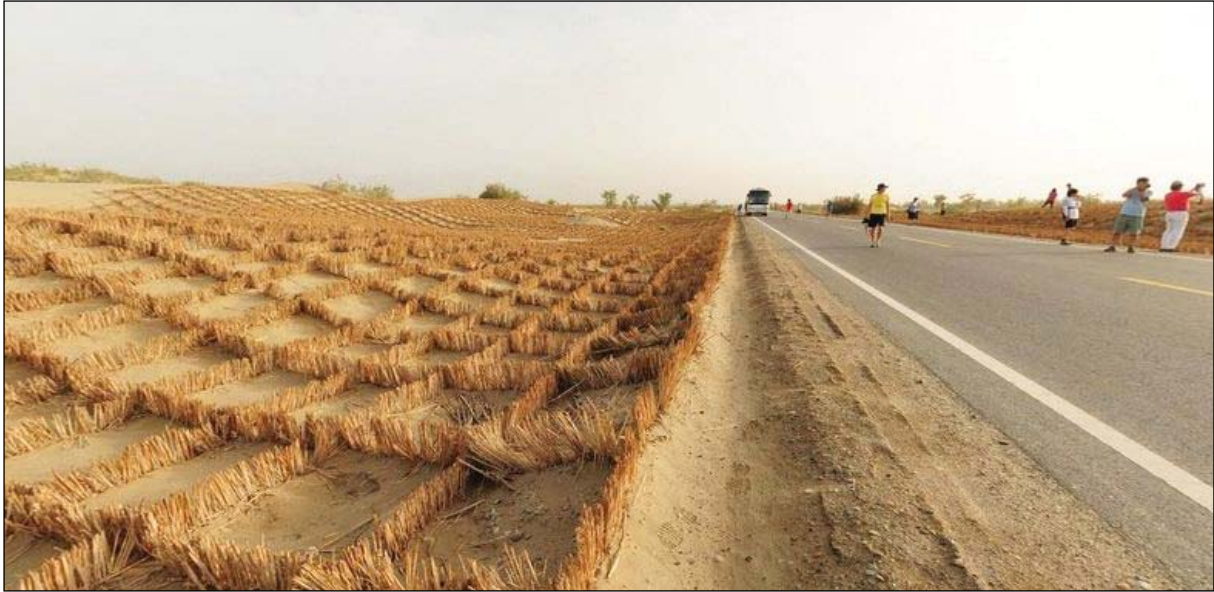
Figure 24. Straw checkerboard technique (DRI 2011) and its application on the Tarim Highway, China (The Tarim Highway, undated).
