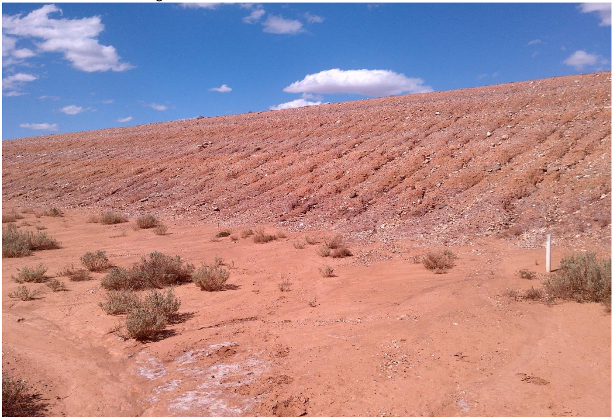
Significant erosion of the Eastern Wall of LRSF by sample location SP30.
