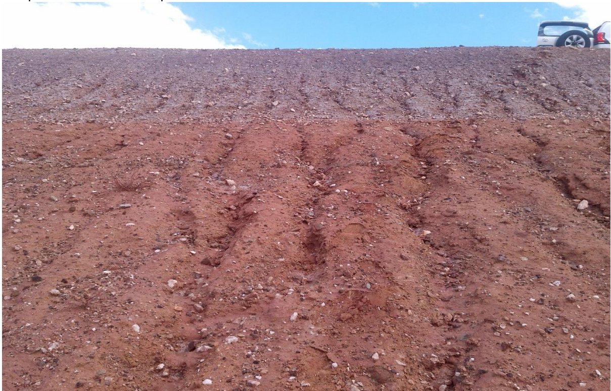
Looking North up to LRSF from sample location SP07. Erosion evident on walls of LRSF at all locations.
