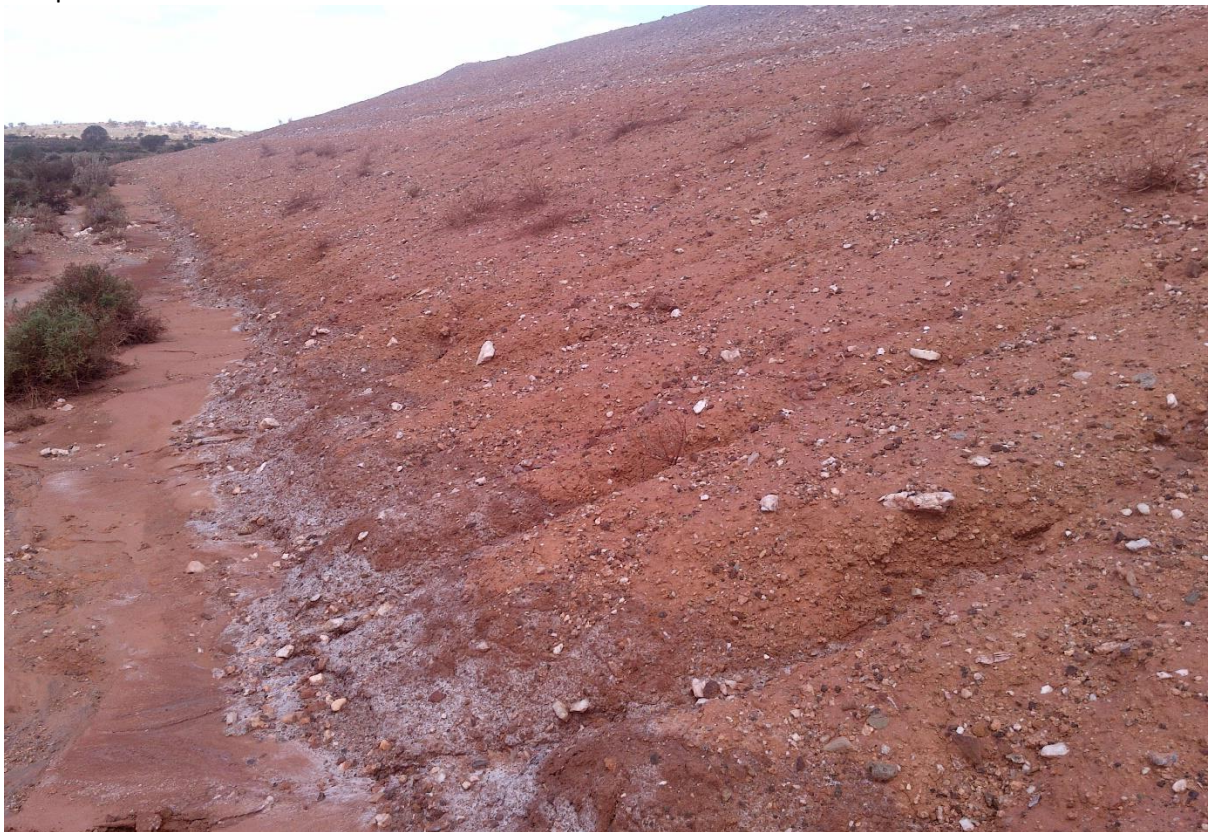
Sample Location SP14 and erosion from North East wall of LRSF.
