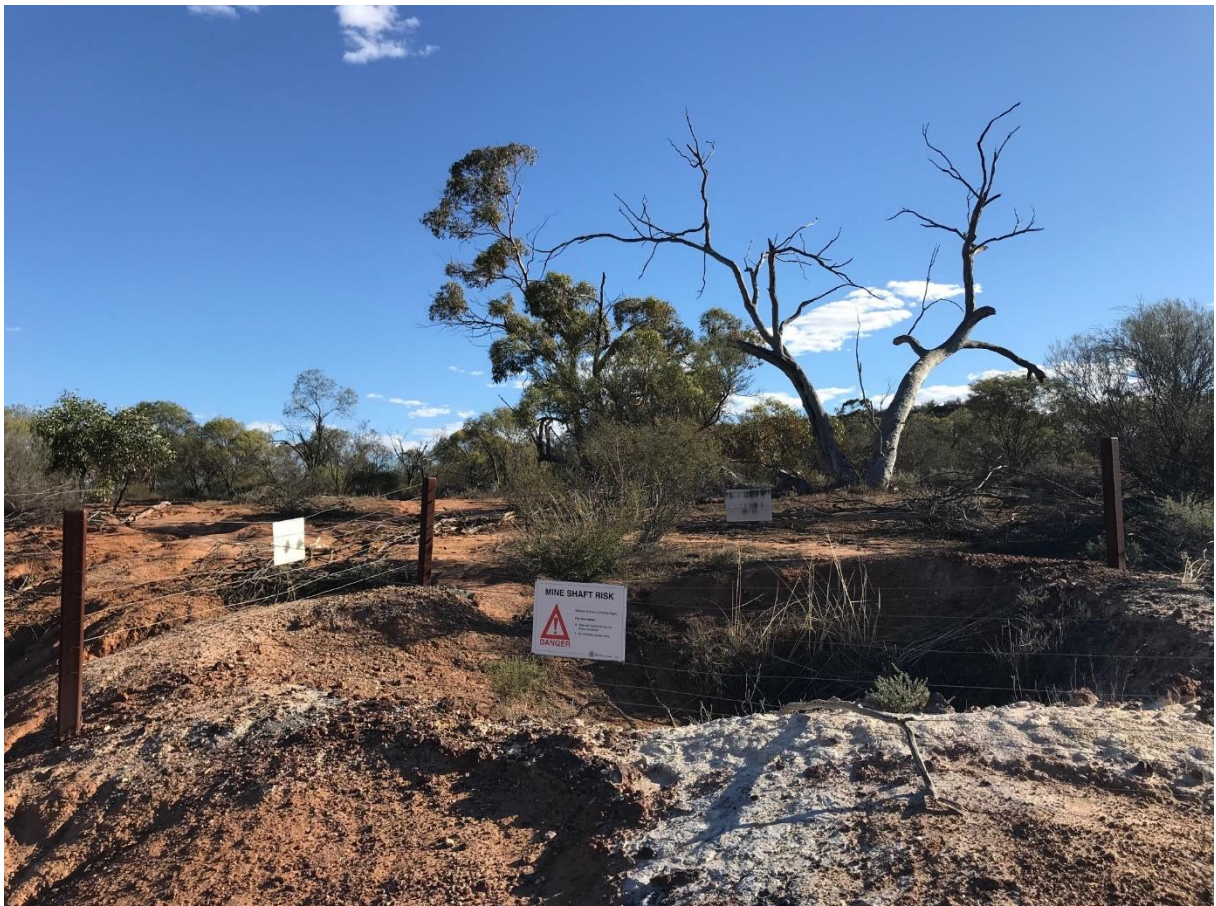
Figure 2: Example of fencing around an abandoned mine shaft (coal mine shafts in Coalseam Conservation Park, Mingenew, WA)
