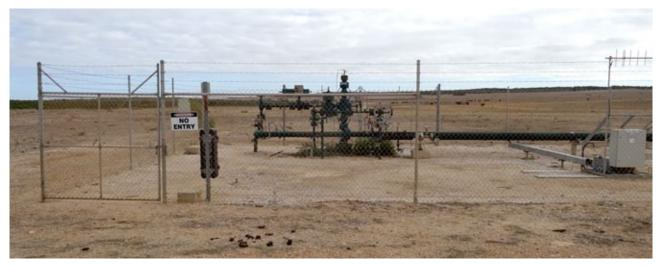
Figure 5: The principal component of a petroleum production well that is visible on the surface is the Christmas tree, an assembly of valves and pipework fitted to the wellhead to control the flow of oil or gas production from the well to a pipeline or a production facility
