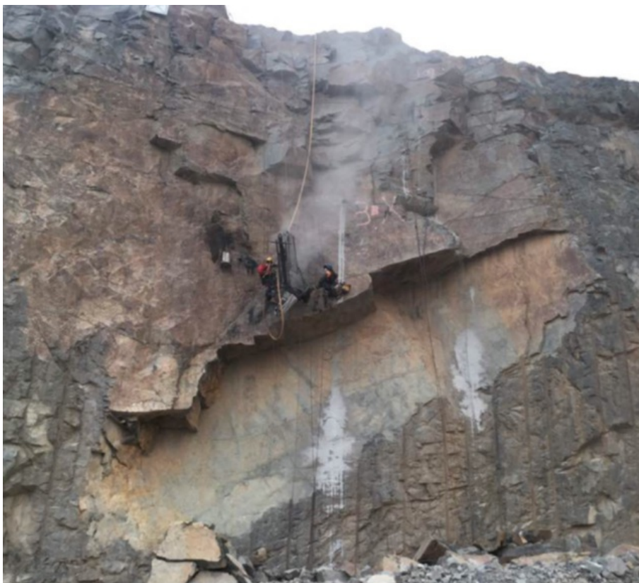
Workers drilling pit wall using rope access
