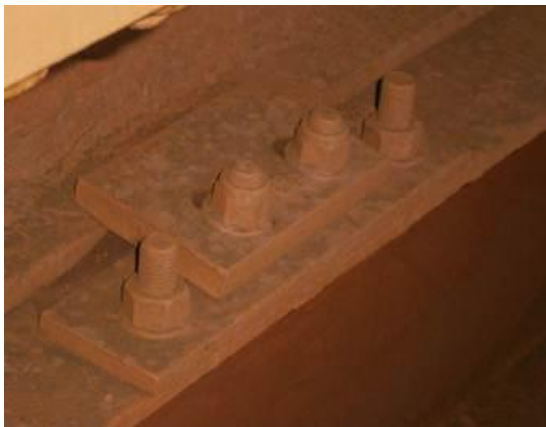
Photographs showing rail clamp as designed by OEM (left) and modified rail clamp (right) with open-ended slots and welded nuts and bolts.
