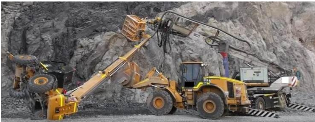
Incident scene showing position of tele-handler and attached work basket.
