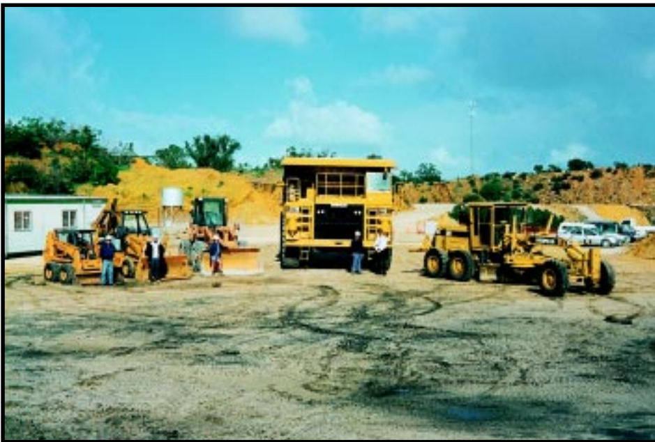
Heavy Equipment Fleet
