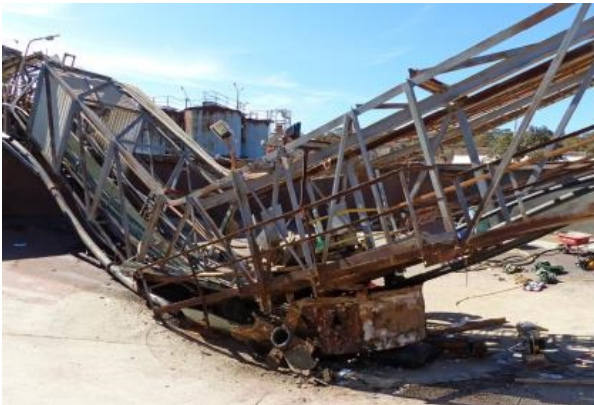
Left. Gantry bridge that failed and collapsed onto the thickener floor. Right. Corroded structural steel angle.
