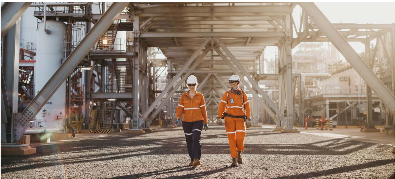
Pluto LNG plant. Image: Woodside Energy Limited.
