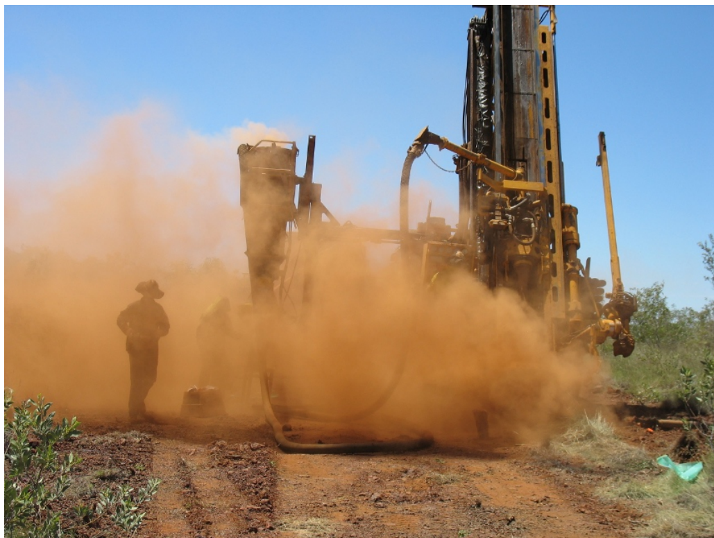
RC drilling with no dust controls in place
