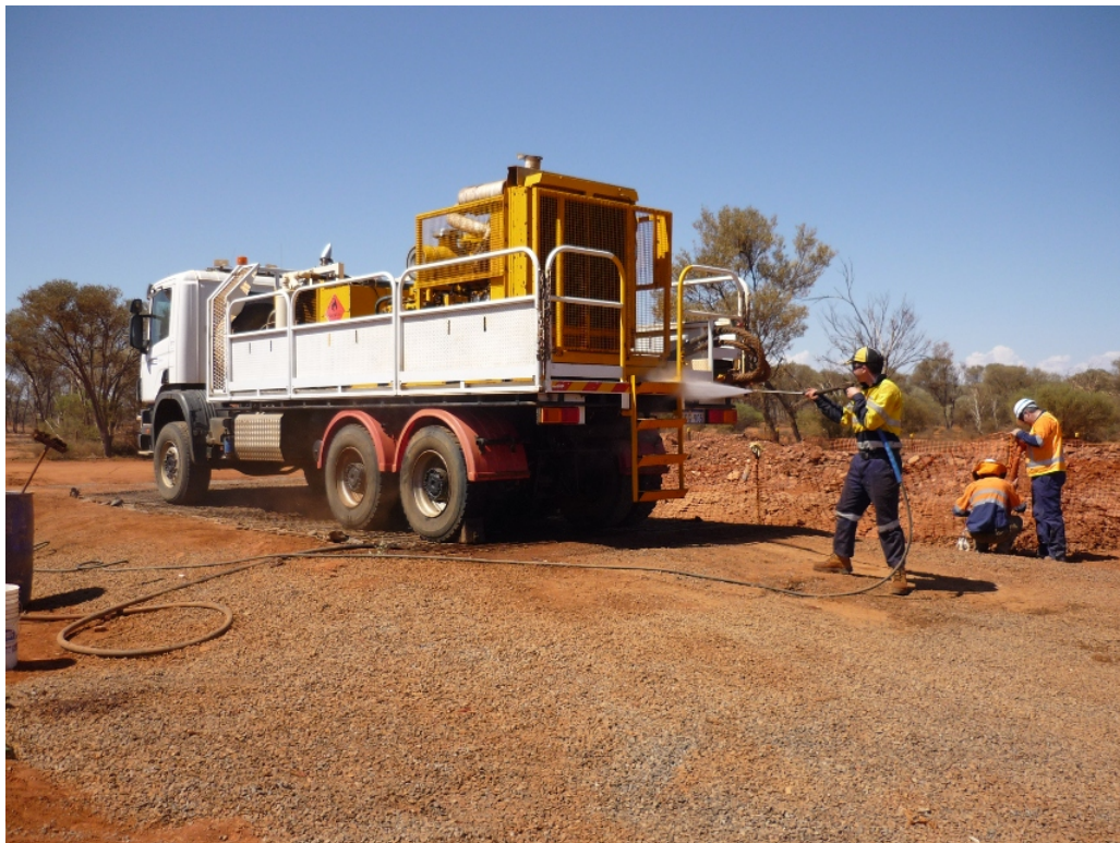
High pressure cleaning of equipment after use. Note large sump to right of picture.
