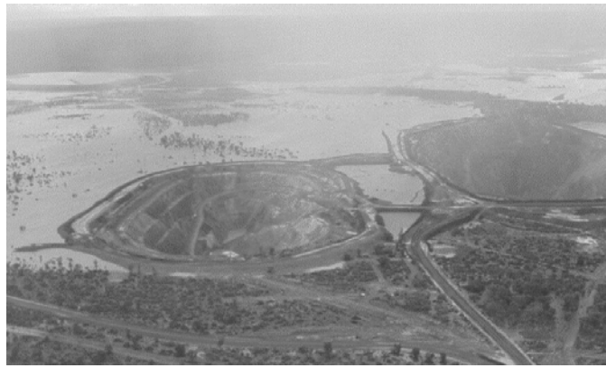
Aerial view of the flood path around the two open pits
