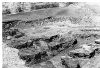
Close up of Stockton open cut in 1949 showing pillars of underground workings. Photograph from 100 years of Collie Coal (Stedman, 1988), reproduced with permission Shire of Collie
