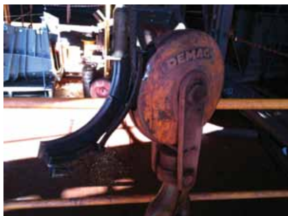
Figure 3 Section of rope guide resting on hook sheave after incident
