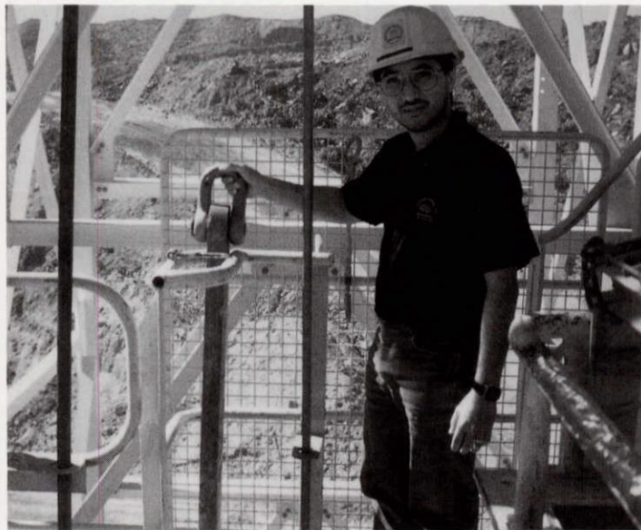
Dominion Mining (Meekatharra) ↑ Storing "J" Hooks on the crusher platform. → Safe storage eliminates trips and slips.
