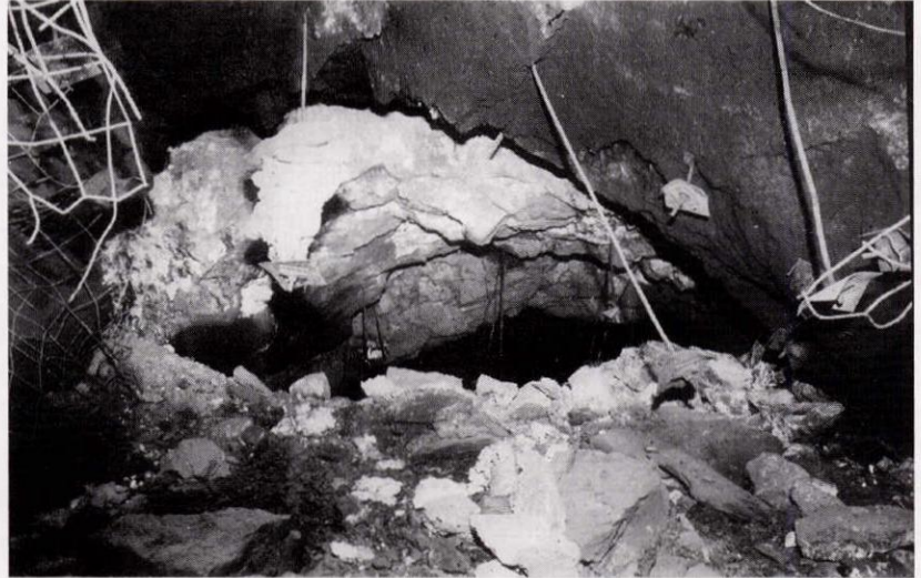
Underground rock fall. Typical cause of crush injuries.
