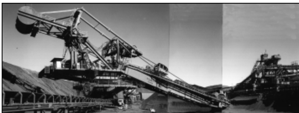
July 1996. The operator was killed when the mast frame collapsed on this reclaimer.
