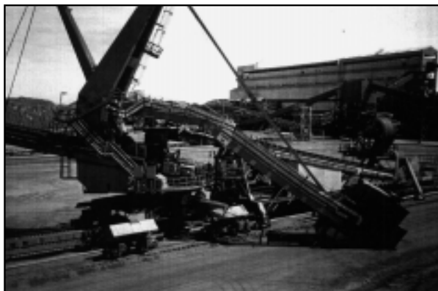
January 1995. A maintenance engineer received serious injuries when the mast frame and counterweight boom collapsed on this stacker.
