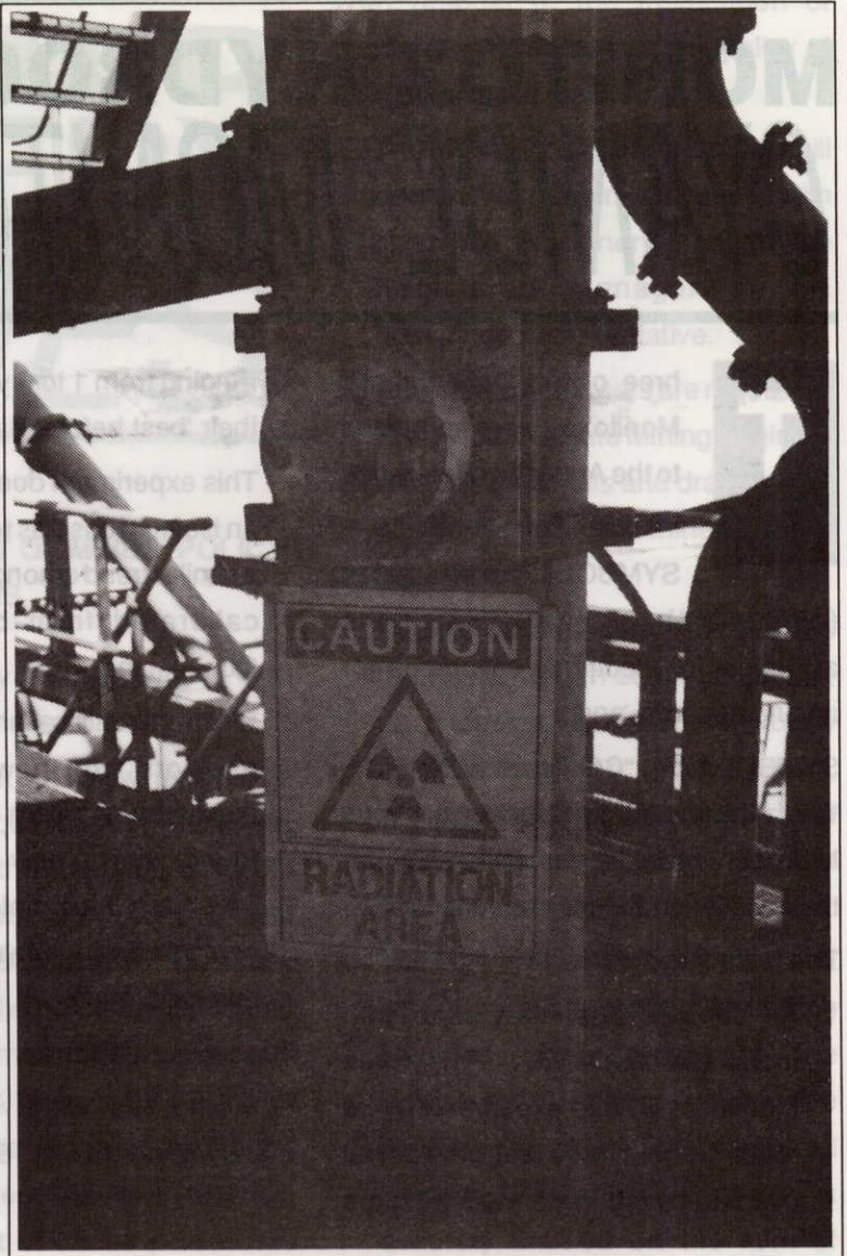
This sign is incorrect. See example below.
