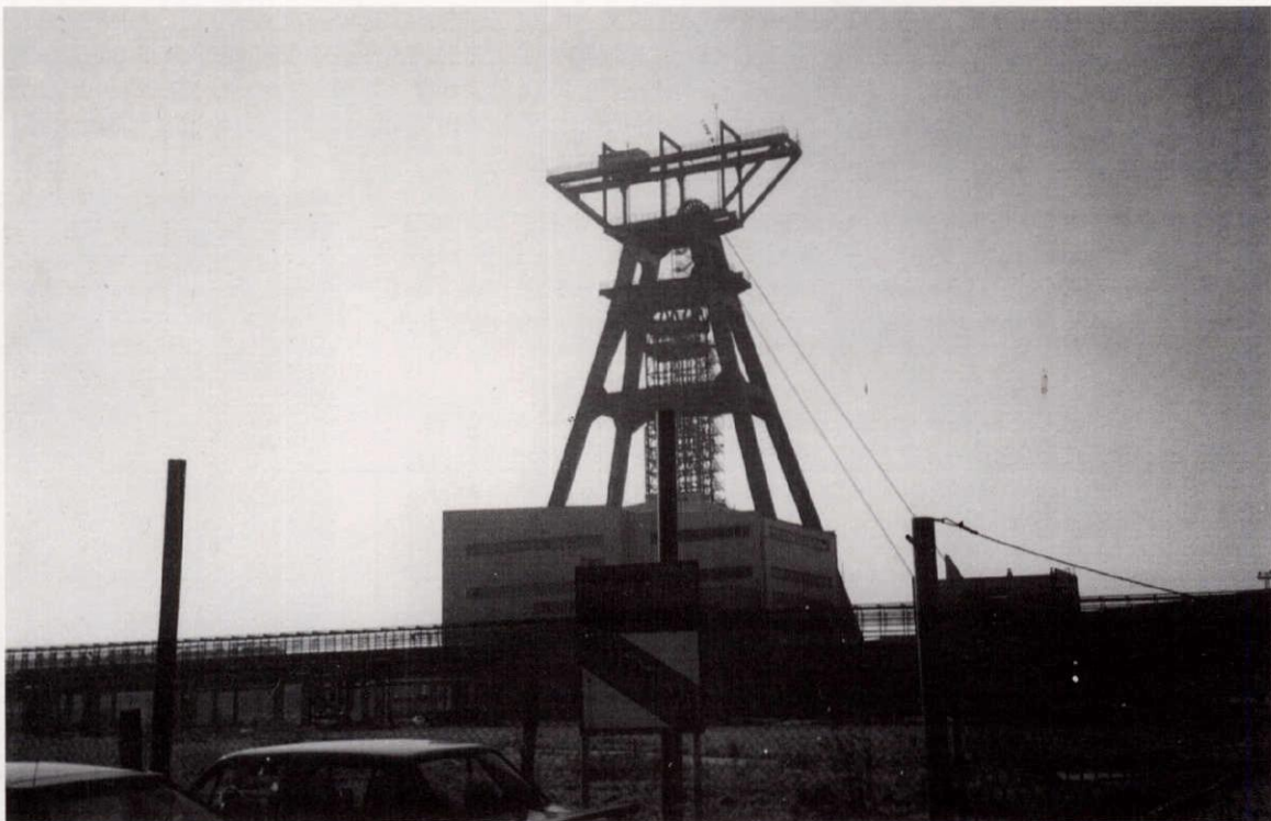
A typical headframe associated with ground mounted friction winders - this one at Ormontowice "Budryk" Coal Mine.
