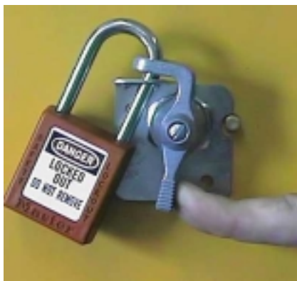
This isolator is now switched on
