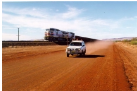
Road built for access to railway assets
