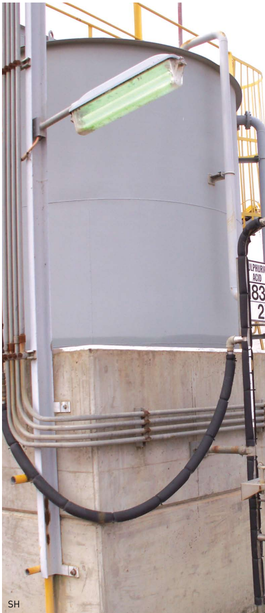
Above: Green light highlights location of emergency shower and eye wash near acid store
