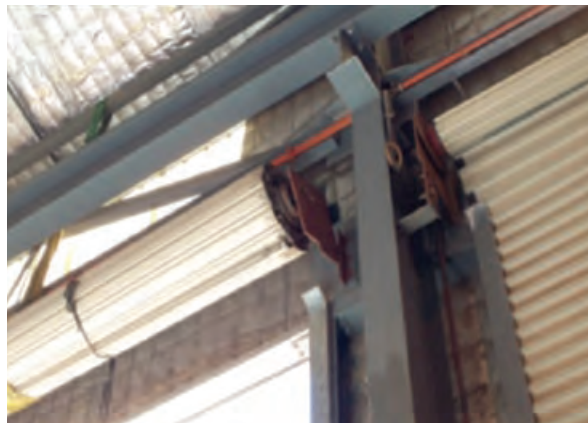
View of non-drive end of roller shutter
