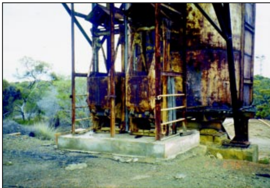
Old mineshaft effectively sealed with concrete capping.
