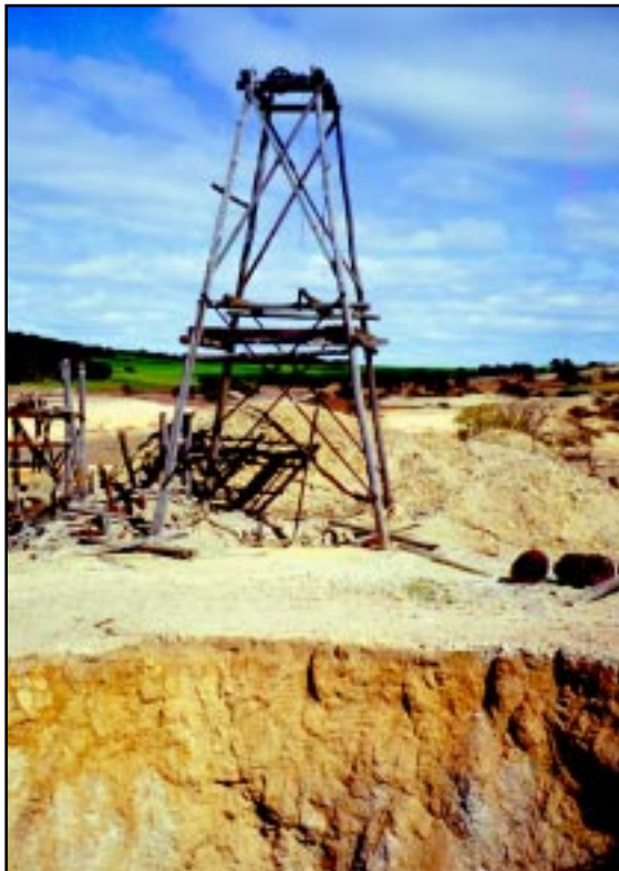
Un-capped shaft with sinkhole in foreground.
