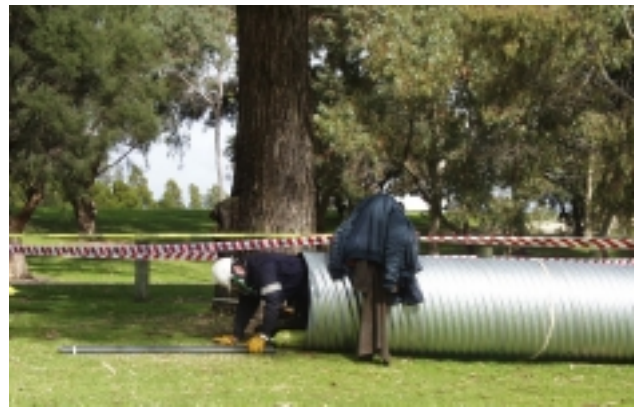
Getting out of a tight spot - Confined Space
