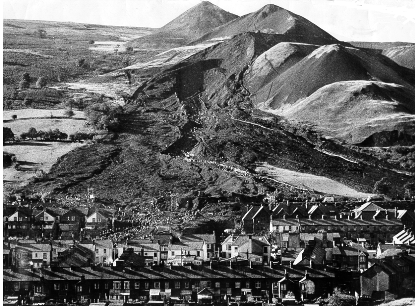
Elevated view of waste dump failure
