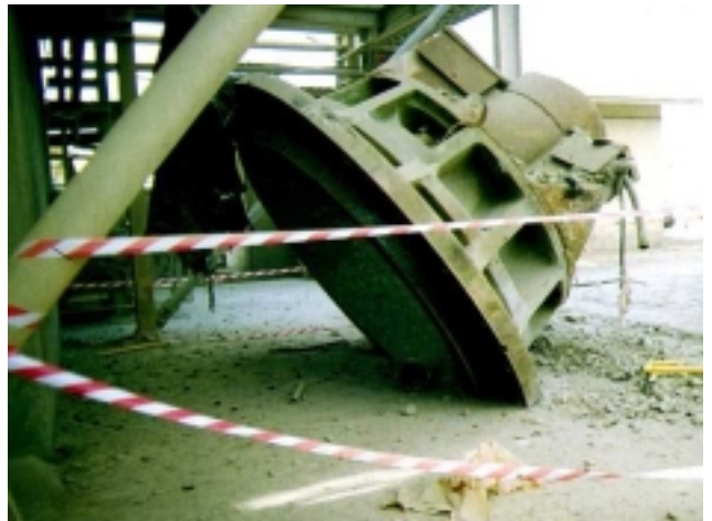
Crusher mantle dropped from crane embedded in concrete floor
