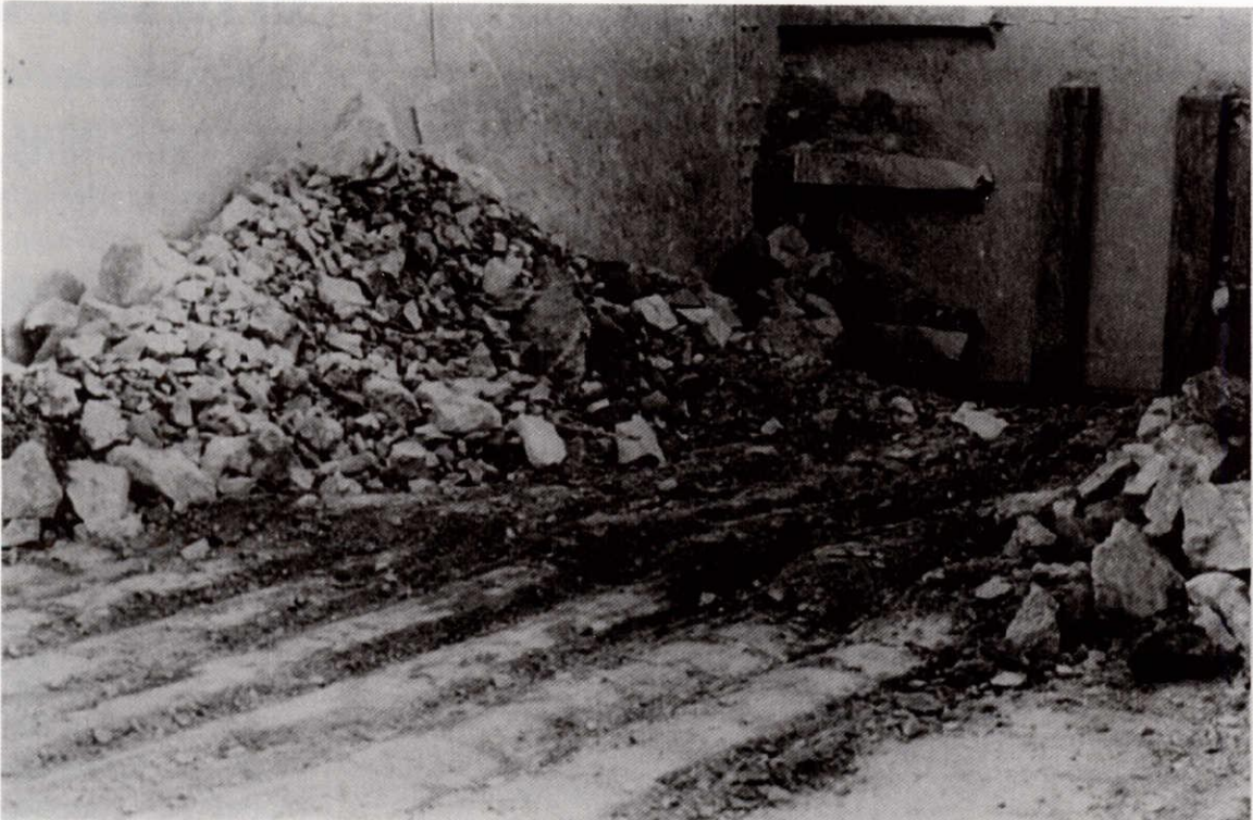
Inadequate barriers on crusher feeder
