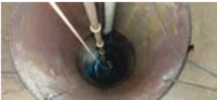
Purpose-built telescoping steel cylinders are welded together to provide a continuous smooth shaft lining
