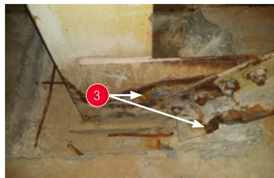
When the concrete around the column is removed it exposes the subsurface corrosion
