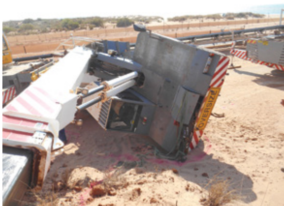
Pick-and-carry crane on its side
