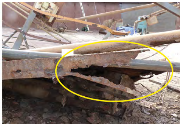
Left: Gantry bridge that failed and collapsed onto the thickener floor. Right: Corroded structural steel angle.
