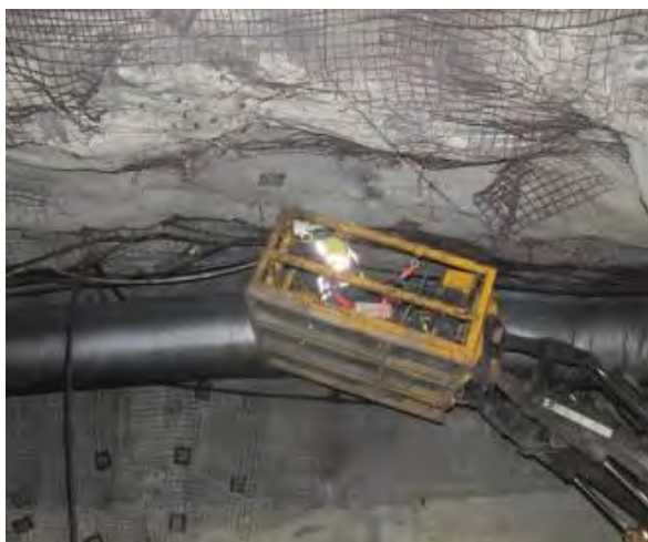
IT work basket in position beneath the backs
