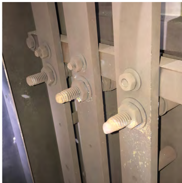
Left: Arc flash damage to the rear compartment of switchboard. Right: Protruding fuse-holder bolts in busbars.
