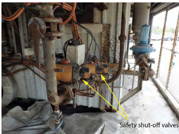
Left: Safety shut-off valves forming part of the burner management system. Right: Damage to boiler
