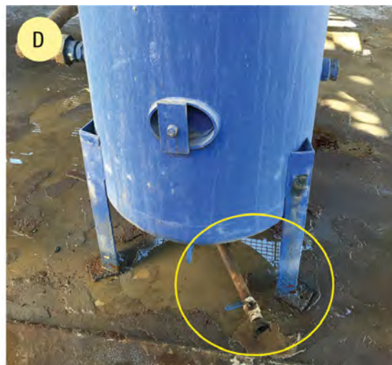
Pressure vessel supports. A. Unanchored vessel containing refrigerated argon gas. B. Air receiver leg anchored to grating only. C. Severe corrosion of a support bracket to an acid elution column (condition of shell unknown). D. Air receiver not bolted down and connection point corroding.
