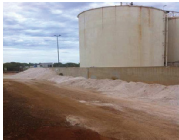
Limestone (piles of pale material) was used to neutralise the second acid spill and support the bund walls
